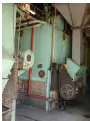
Plate P112: Building TA21 - typical boiler which is insulated with SMF. Note: brick support walls contain asbestos rope caulking
