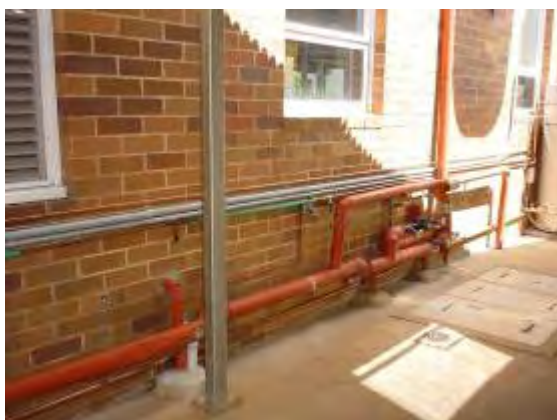
Plate P51: Building TA15 - hot water pipework along east side wall which is insulated with SMF
