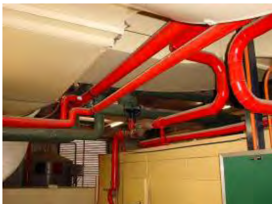
Plate P87: Building TA20 - hot water tanks to main roof level plantroom which are insulated with either asbestos or SMF
