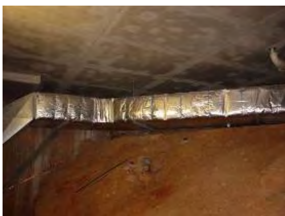
Plate P101: Building TA20 - air conditioning ductwork to foundation space which is insulated with SMF
