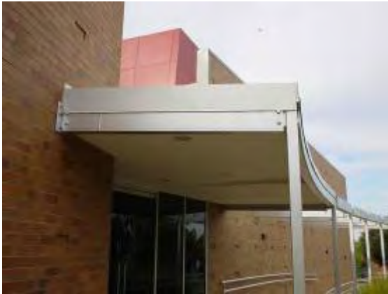
Plate P157: Building TA35 - fibrous cement ceiling linings to west side awning which do not contain asbestos
