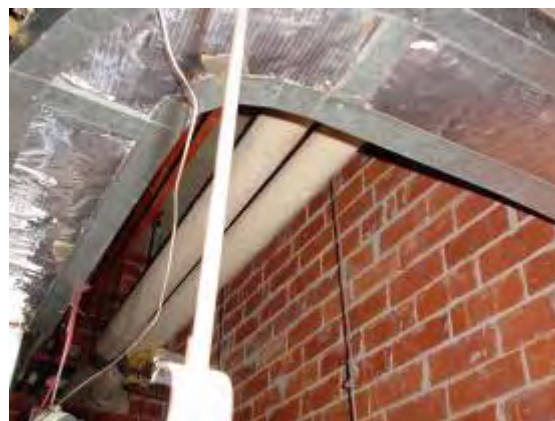
Plate P94: Building TA20 - asbestos lagged pipework to ceiling space and air conditioning ductwork which is insulated with SMF
