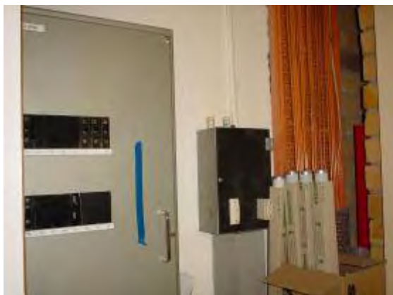
Plate P91: Building TA20 - asbestos containing backing board to typical electrical cupboard
