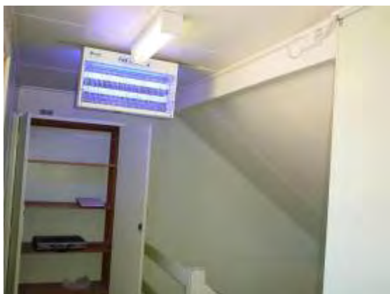
Plate P53: Building TA15 - asbestos cement internal wall and ceiling linings to south west access stair
