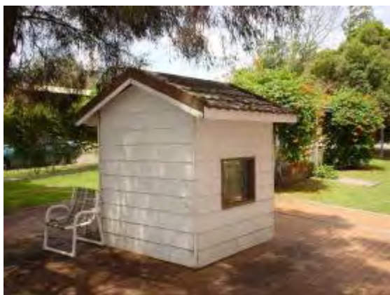
Plate P71: Building TA18 - fibrous cement weatherboards to cubby house which do not contain asbestos
