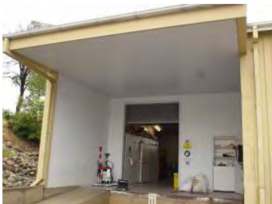
Plate P119: Building TA23 - fibrous cement wall and ceiling linings to contaminated waste dock which do not contain asbestos
