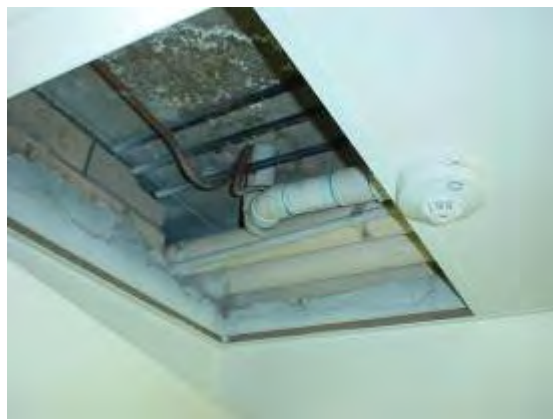
Plate P134: Building TA26 - asbestos lagged pipework in ceiling space
