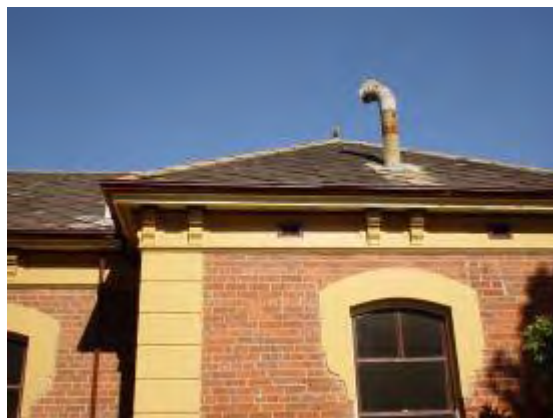
Plate P76: Building TA19 - asbestos cement shingle tiles to south east projecting wing
