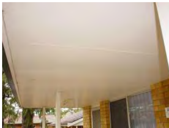
Plate P20: Building TA09 - asbestos cement ceiling linings to south side verandah
