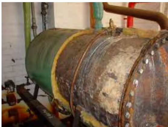
Plate P73: Building TA18 - boilers to south side boiler room which are insulated with SMF
