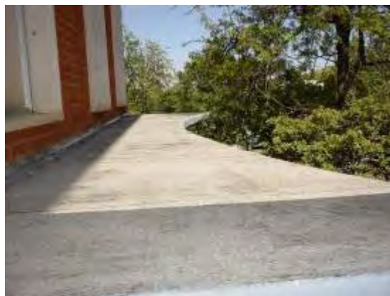
Plate P128: Building TA26 - typical bituminous roofing membrane to concrete awning which contains asbestos
