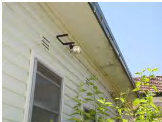
Plate P40: Building TA13 - asbestos cement eaves linings to south side of west wing
