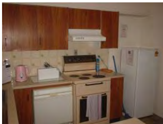
Plate P10: Building TA05 - asbestos cement wall linings behind wall tiles and cupboards to kitchen
