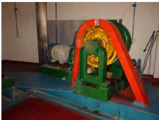
Plate P85: Building TA20 - lift motor to main roof level lift motor room which is likely to contain asbestos brake shoes
