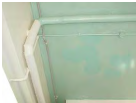
Plate P56: Building TA15 - asbestos lagged pipework to main kitchen area
