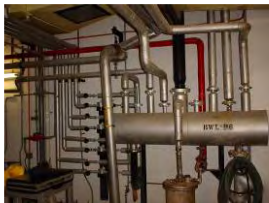
Plate P96: Building TA20 - typical asbestos lagged pipework and manifold to lower ground floor plant area
