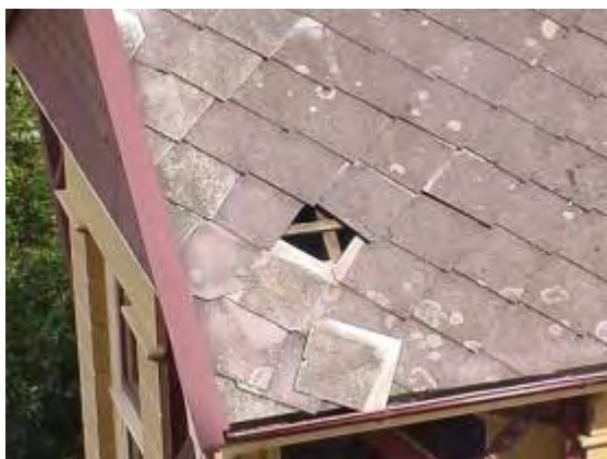
Plate P77: Building TA19 - dislodged asbestos cement shingle tiles to south east project wing
