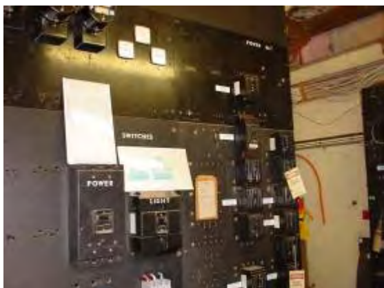
Plate P83: Building TA19 - asbestos containing backing boards to main electrical room
