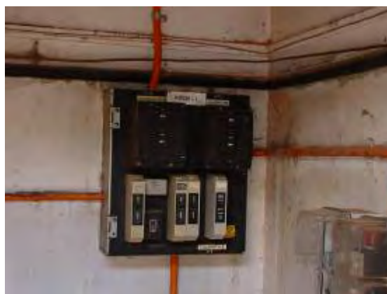
Plate P52: Building TA15 - asbestos containing electrical backing board to east side Compressor Enclosure
