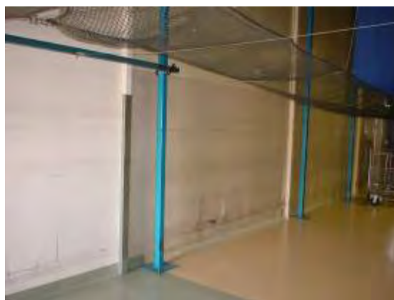
Plate P114: Building TA21 - fibrous cement walling to Sorting Dock (outer portion) which does not contain asbestos
