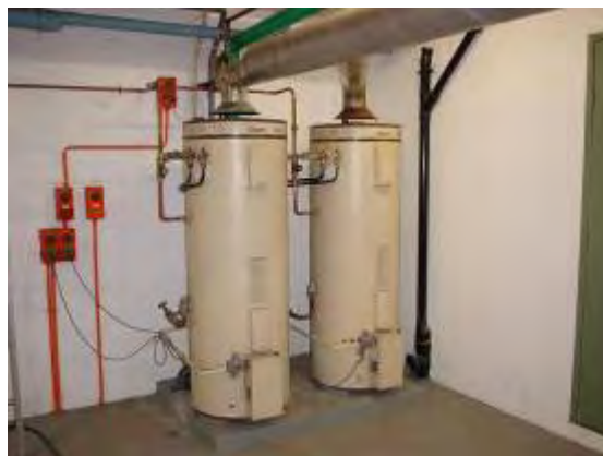
Plate P28: Building TA11 - hot water units to basement level boiler room which are insulated with SMF
