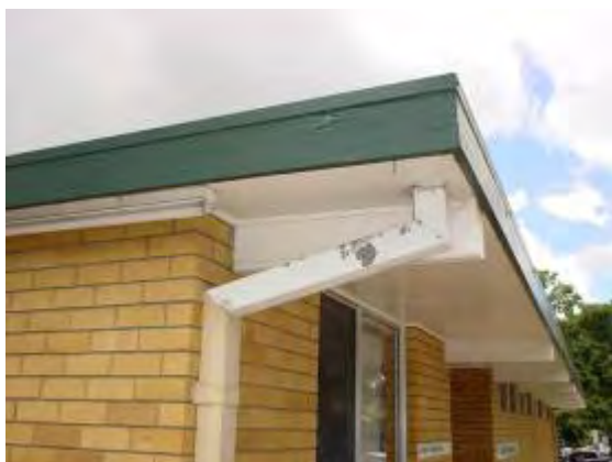
Plate P29: Building TA11 - asbestos cement eaves linings to projecting north side wing
