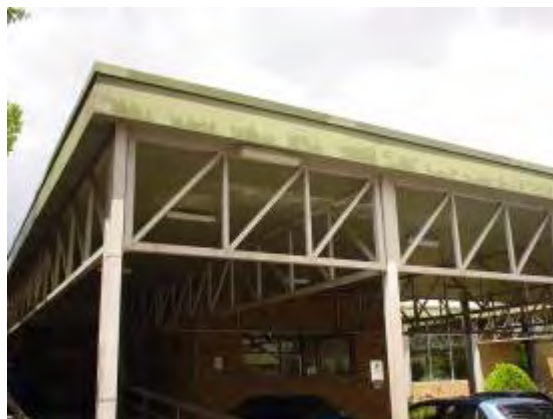
Plate P26: Building TA11 - fibrous cement ceiling linings to large north west parking area which do not contain asbestos
