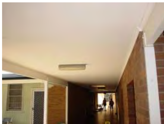
Plate P48: Building TA15 - ceiling linings to east side covered way which do not contain asbestos
