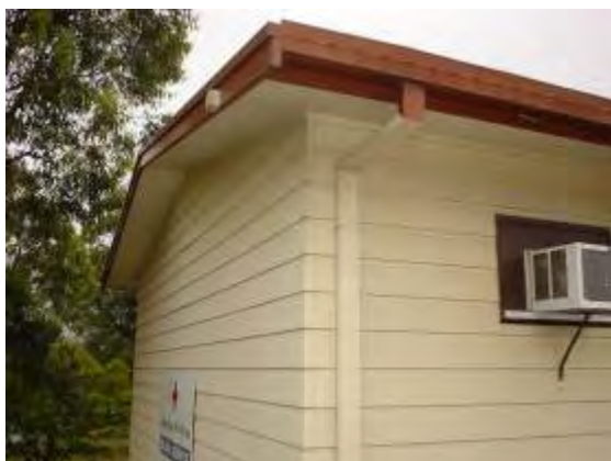
Plate P125: Building TA25 - fibrous cement walling and eaves to eastern portion which do not contain asbestos
