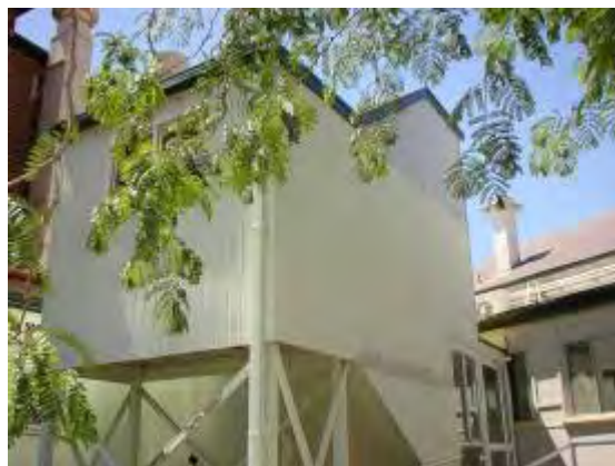
Plate P50: Building TA15 - asbestos cement walling to south west access stair
