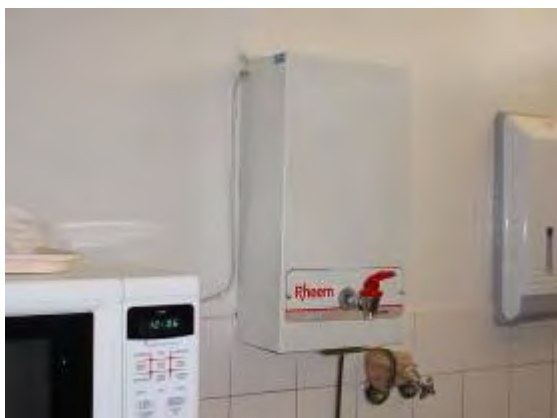
Plate P107: Building TA21 - boiling water unit to staff lunchroom which is insulated with SMF
