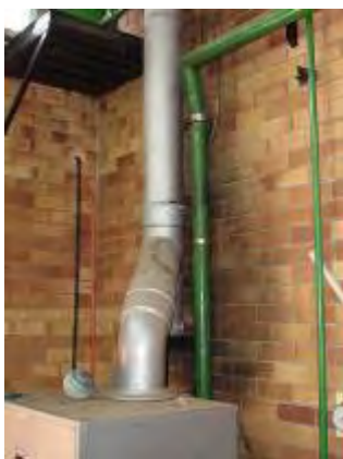
Plate P147: Building TA29 - asbestos cement flue to boiler
