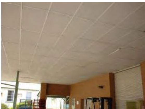
Plate P65: Building TA16 - ceiling linings to main south side dock which do not contain asbestos
