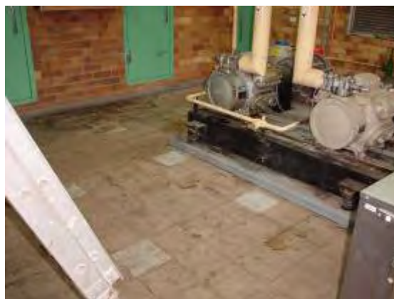
Plate P144: Building TA29 - typical vinyl floor tiles which do not contain asbestos
