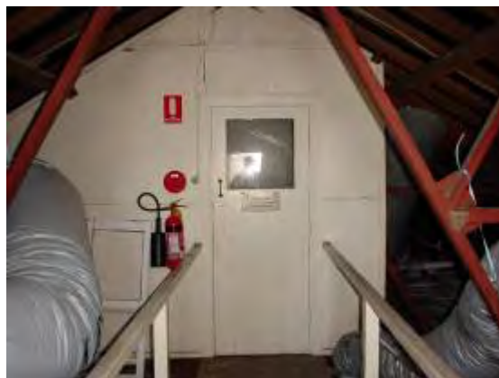
Plate P62: Building TA15 - lift motor room in roof space which is likely to contain asbestos backing boards/materials
