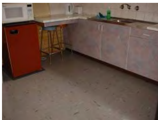
Plate P22: Building TA09 - vinyl floor tiles to kitchen which do not contain asbestos
