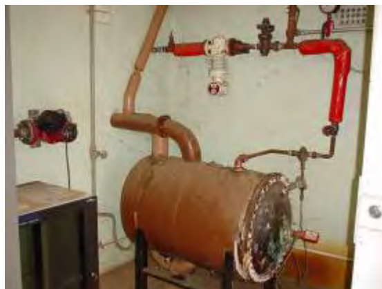
Plate P16: Building TA07 - boiler and pipework to south west boiler room which are insulated with SMF. Note: asbestos gaskets to flanged joints presumed.
