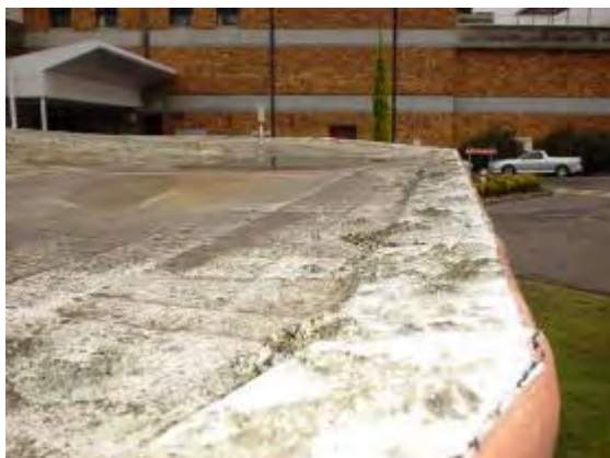
Plate P123: Building TA25 - asbestos containing bituminous membrane to roof of original western portion of building
