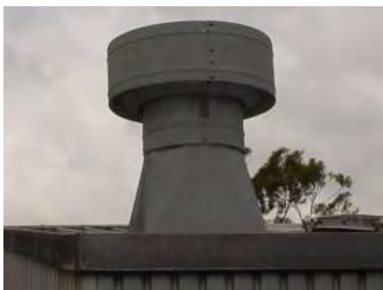
Plate P149: Building TA30 - roof vent which is possibly finished with asbestos "Galbestos" paint
