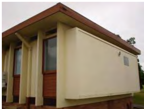
Plate P116: Building TA22 - fibrous cement wall and eaves linings which do not contain asbestos
