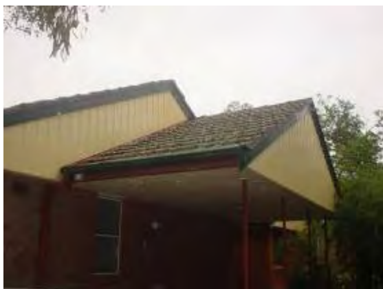
Plate P9: Building TA05 - asbestos cement linings to roof gables, eaves and ceiling of carport
