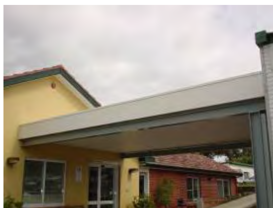
Plate P46: Building TA14 - fibrous cement fascia and ceiling linings to entry porte cochere which do not contain asbestos
