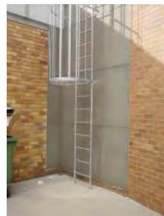
Plate P156: Building TA35 - fibrous cement walling at north end which does not contain asbestos
