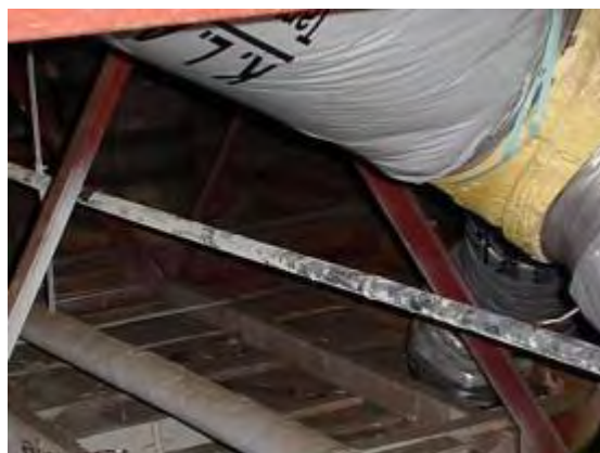
Plate P60: Building TA15 - air conditioning ductwork in roof space which is insulated with SMF and residue to pipework which does not contain asbestos
