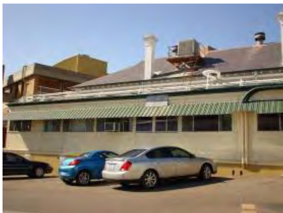
Plate P79: Building TA19 - asbestos cement walling to verandah, north side east end
