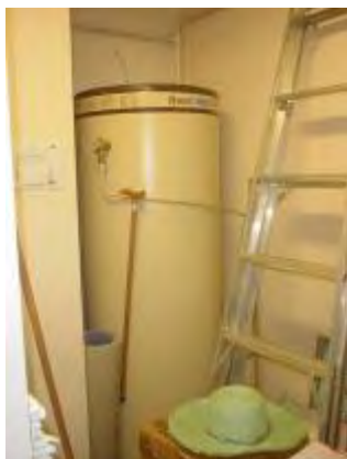
Plate P3: Building TA01 - hot water unit to Cleaners Linen/Store which is insulated with SMF.
