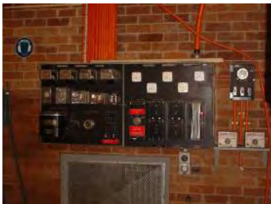
Plate P109: Building TA21 - asbestos containing electrical boards to Engineering Workshop area
