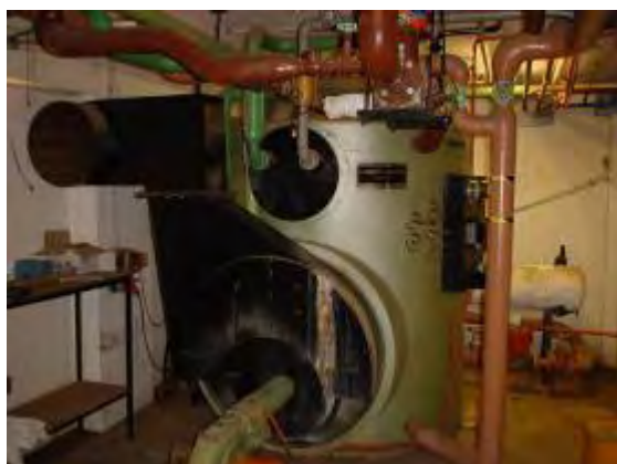
Plate P137: Building TA26 - boiler which is most likely insulated with SFM and which contains asbestos gaskets
