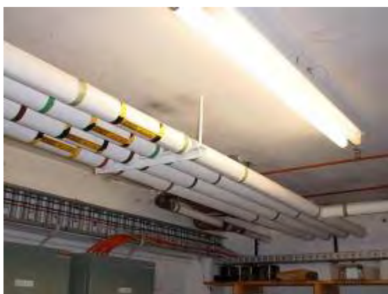
Plate P135: Building TA26 - asbestos lagged pipework to plant/boiler room
