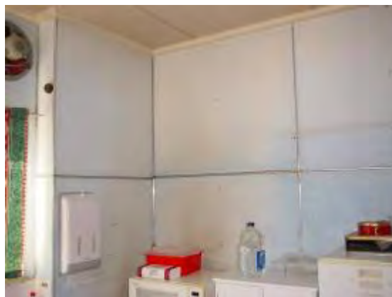
Plate P82: Building TA19 - asbestos cement wall and ceiling linings to north east kitchen/lunchroom
