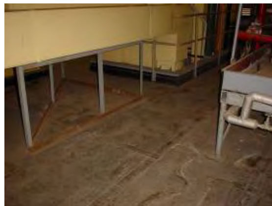
Plate P86: Building TA20 - asbestos containing membrane to floor of main roof level plantroom
