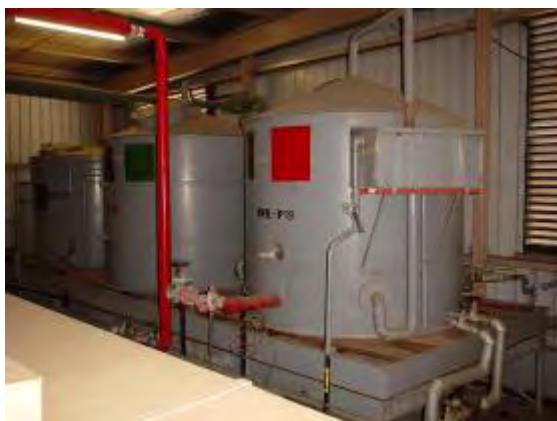
Plate P87: Building TA20 - hot water tanks to main roof level plantroom which are insulated with either asbestos or SMF
