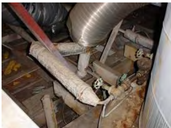
Plate P57: Building TA15 - hot water unit to south end hot water cupboard which is insulated with SMF
