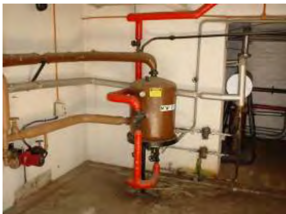
Plate P81: Building TA19 - calorifier and pipework to east end boiler room which are insulated with asbestos lagging
