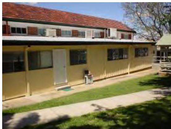
Plate P38: Building TA13 - profiled asbestos cement wall linings at north west corner and flat wall linings which do not contain asbestos
