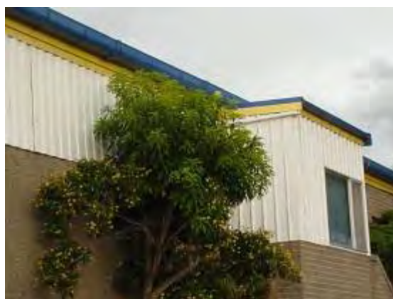
Plate P12: Building TA06 - typical asbestos cement wall linings and eaves gutters
