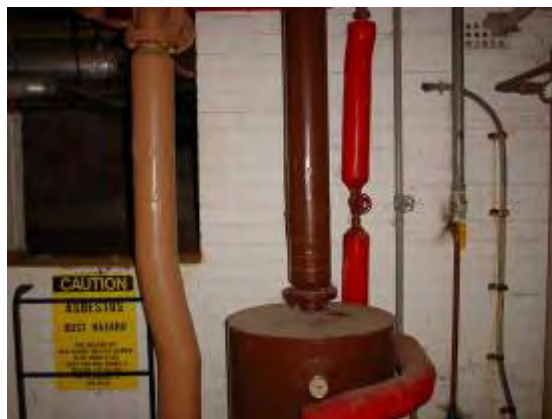
Plate P80: Building TA19 - boiler and pipework to east end boiler room which are insulated with asbestos lagging
