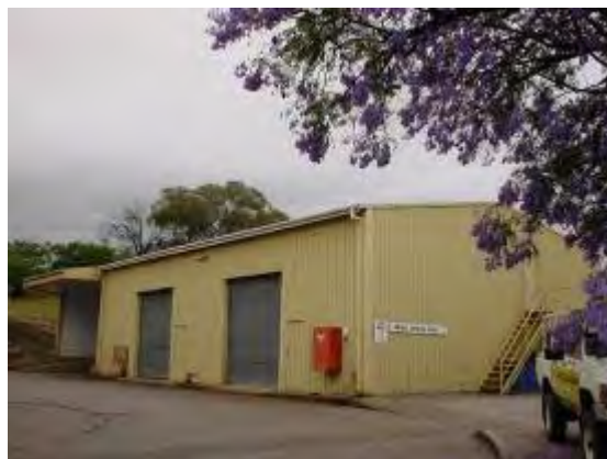
Plate P116: Building TA22 - fibrous cement wall and eaves linings which do not contain asbestos
