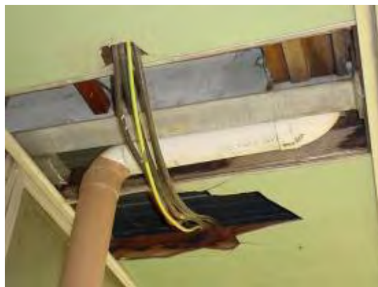
Plate P104: Building TA21 - damaged asbestos cement ceiling lining to breezeway adjacent workshop offices
