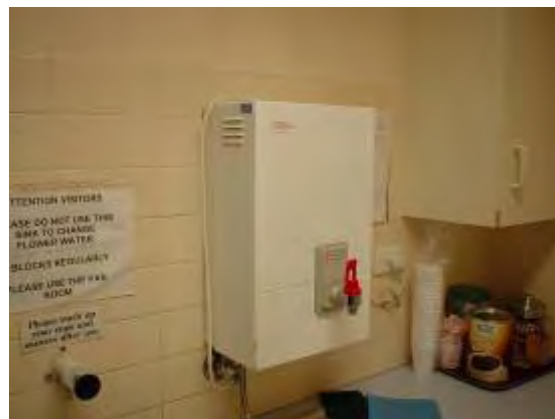
Plate P92: Building TA20 - typical boiling water unit which is insulated with SMF
