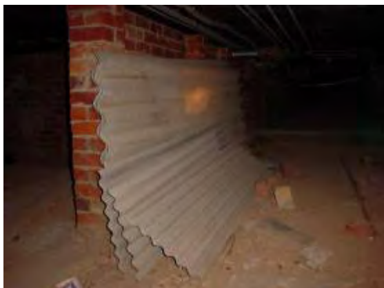
Plate P33: Building TA12 - stored asbestos cement sheeting in foundation space
