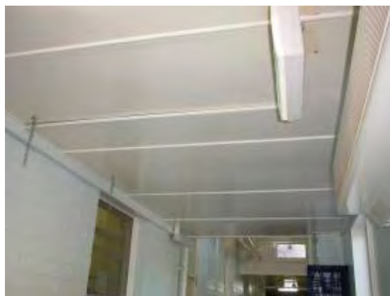
Plate P52: Building TA15 - asbestos containing electrical backing board to east side Compressor Enclosure
