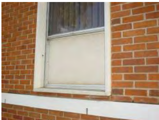
Plate P127: Building TA26 - typical asbestos cement window spandrel panel. Note: putty to window frames also contains asbestos
