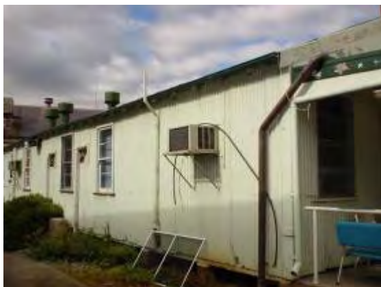
Plate P67: Building TA17 - asbestos cement wall linings to east side of building
