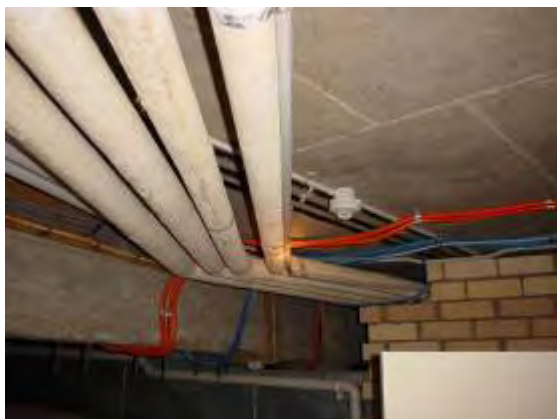
Plate P133: Building TA26 - asbestos lagged pipework in foundation space
