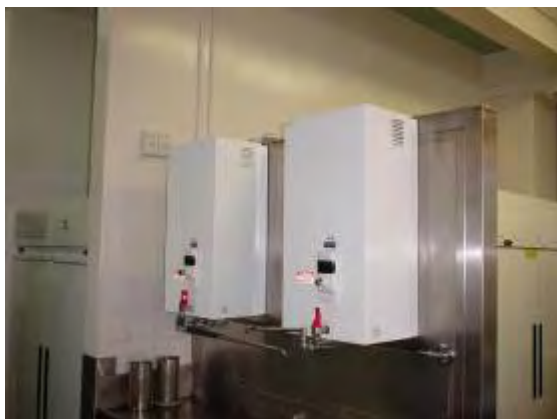
Plate P55: Building TA15 - boiling water units to main kitchen area which are insulated with SMF
