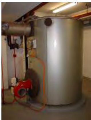
Plate P27: Building TA11 - boiler to basement level boiler room which is insulated with SMF
