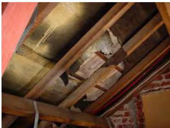
Plate P61: Building TA15 - sarking to underside of roof tiles which does not contain asbestos
