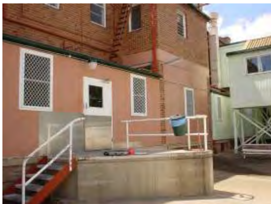
Plate P49: Building TA15 - flat fibrous cement walling (pink and green) to west side which does not contain asbestos
