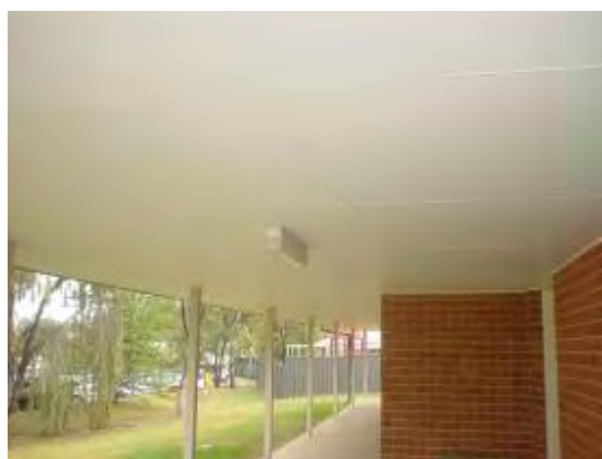
Plate P154: Building TA34 - fibrous cement ceiling linings to south side verandah which do not contain asbestos
