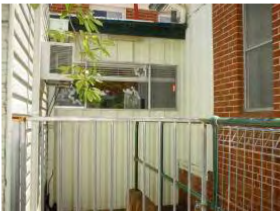
Plate P39: Building TA13 - asbestos cement wall linings to south side recess
