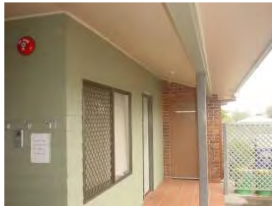
Plate P2: Building TA01 - typical eaves, porch ceiling and wall linings which do not contain asbestos.
