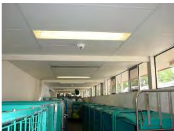
Plate P113: Building TA21 - ceiling tiles to Clean Store which do not contain asbestos
