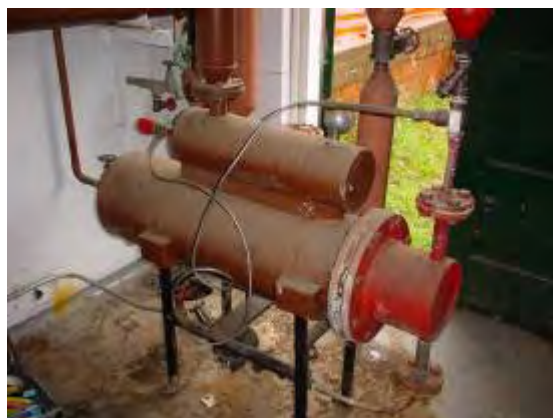
Plate P36: Building TA12 - calorifier to south east boiler room which is insulated with either asbestos or SMF
