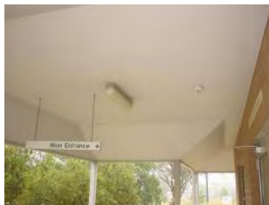
Plate P6: Building TA03 - typical eaves and porch ceiling linings which do not contain asbestos
