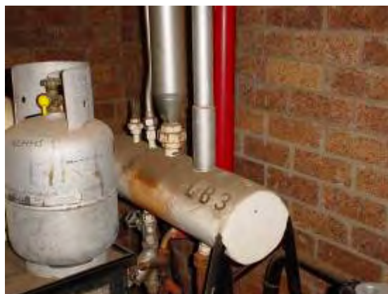
Plate P108: Building TA21 - asbestos lagged manifold to west end storeroom, Engineering Workshop area
