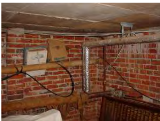
Plate P17: Building TA07 - typical pipework to foundations which is insulated with SMF
