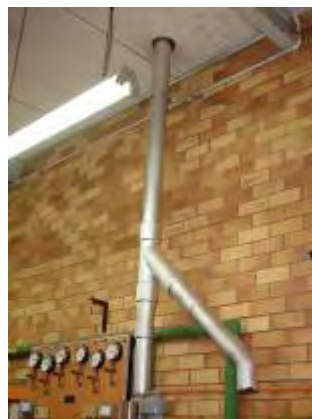
Plate P146: Building TA29 - asbestos cement flue to gas hot water unit. Note: asbestos cement ceiling linings
