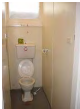
Plate P42: Building TA13 - asbestos cement wall linings to south end toilet
