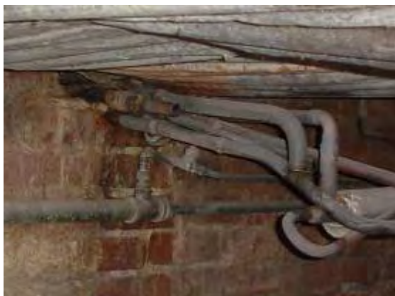
Plate P63: Building TA15 - asbestos rope insulation to portions of pipework in foundations spaces
