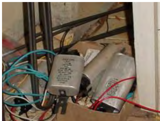
Plate P58: Building TA15 - redundant PCB containing fluorescent light capacitors to floor of south end hot water cupboard
