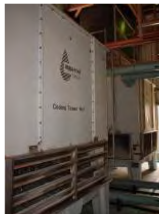
Plate P90: Building TA20 - fibreglass cooling tower to main roof level plantroom which contain SMF
