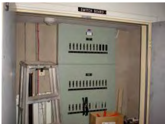
Plate P131: Building TA26 - electrical cabinet which is likely to contain asbestos backing boards or mounting strips
