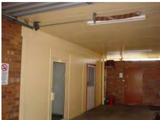
Plate P117: Building TA22 - asbestos cement walling to vehicle dock. Note: ceiling does not contain asbestos
