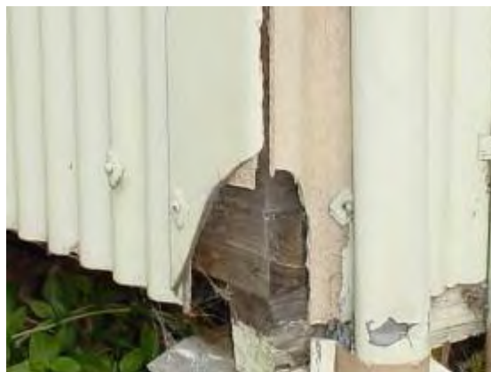
Plate P68: Building TA17 - damaged asbestos cement wall linings at south east corner
