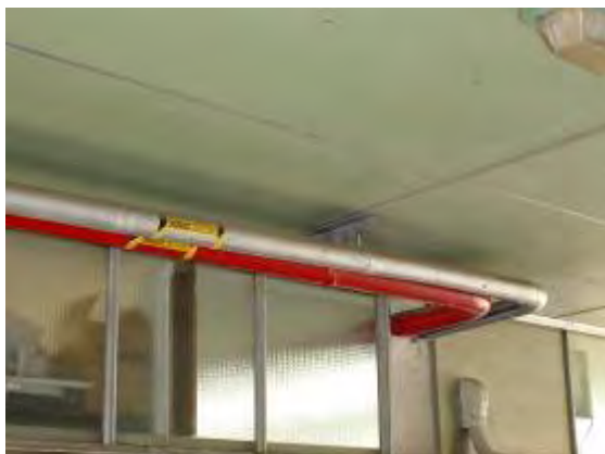
Plate P105: Building TA21 - external asbestos lagged pipework to breezeway, south wing. Note: asbestos cement ceiling linings
