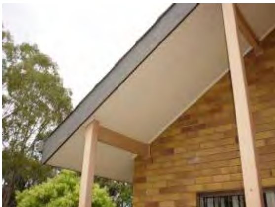
Plate P139: Building TA27 - fibrous cement eaves and porch ceiling linings which do not contain asbestos
