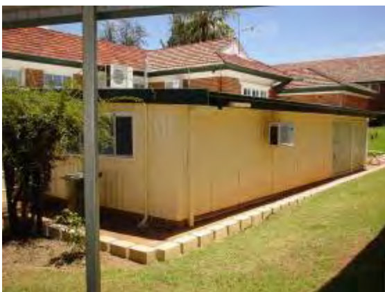
Plate P41: Building TA13 - asbestos cement wall linings to east side extension
