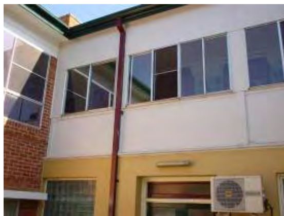
Plate P78: Building TA19 - asbestos cement upper and lower walling to verandah, south side, west end
