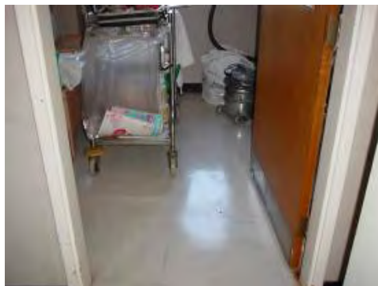
Plate P130: Building TA26 - asbestos containing vinyl floor tiles to second floor utility room
