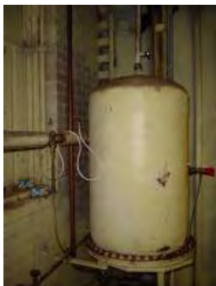
Plate P57: Building TA15 - hot water unit to south end hot water cupboard which is insulated with SMF
