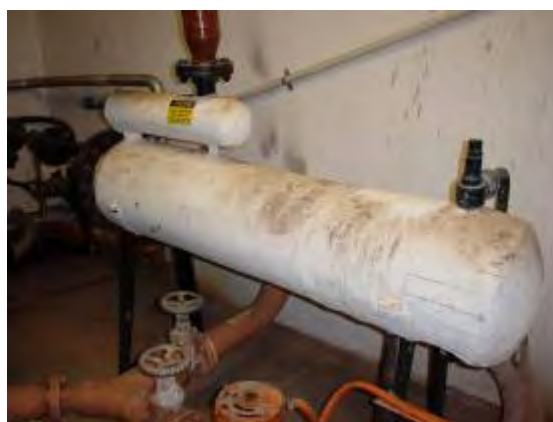
Plate P136: Building TA26 - asbestos lagged calorifier to plant/boiler room
