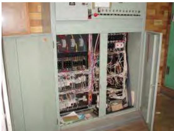
Plate P145: Building TA29 - asbestos containing backing boards to main electrical control cabinets
