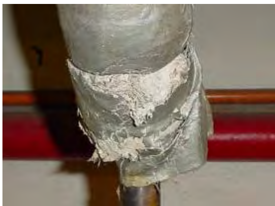
Plate P99: Building TA20 - damaged/exposed asbestos pipe lagging in basement plant area
