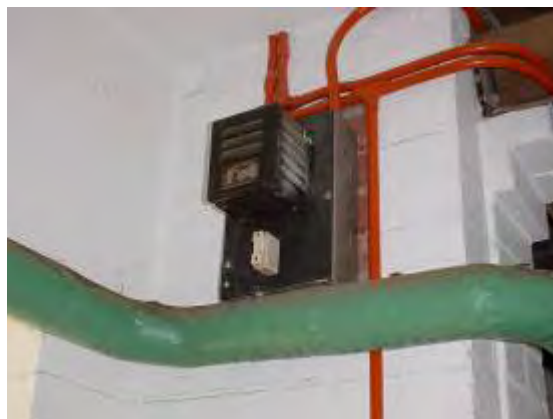
Plate P74: Building TA18 - asbestos containing electrical board to south side boiler room
