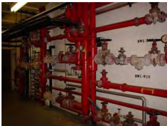
Plate P97: Building TA20 - typical asbestos lagged pipework to lower ground floor plant area
