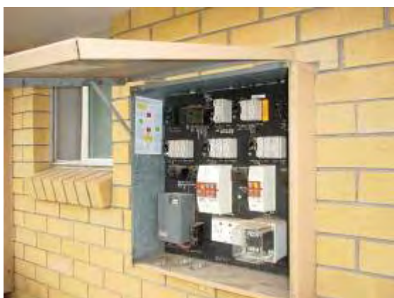
Plate P21: Building TA09 - asbestos containing backing board to north side electrical cabinet
