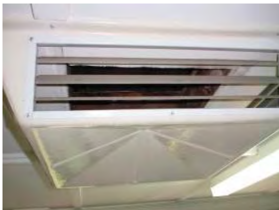
Plate P121: Building TA24 - exposed edges to asbestos cement ceiling linings to north side verandah at vent
